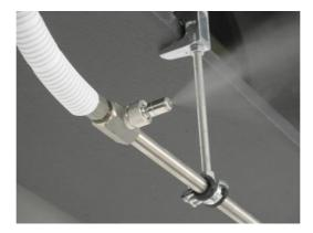
Joints are used in areas where nozzle spray may be hampered (eg, by obstructions such as lamps, chains, cables, etc.). This joint allows a nozzle to be turned by 30° in any direction, provided it is switched off. Spray is then not impeded by the obstruction. A feature of the joint is that in any position on all components it can handle the operating pressure of 80 bar. Alternatively, nozzles can be replaced by a blind plug.
